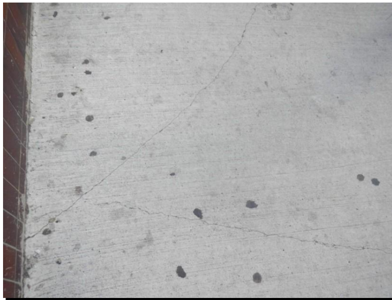
Concrete with multiple hairline cracks
