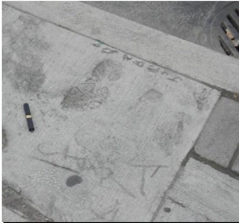
Concrete containing undesirable impressions
