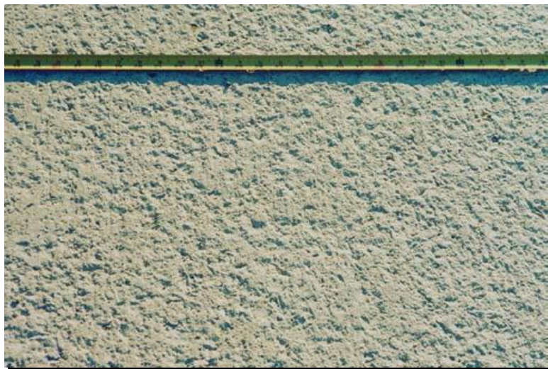
Concrete damaged by rain
